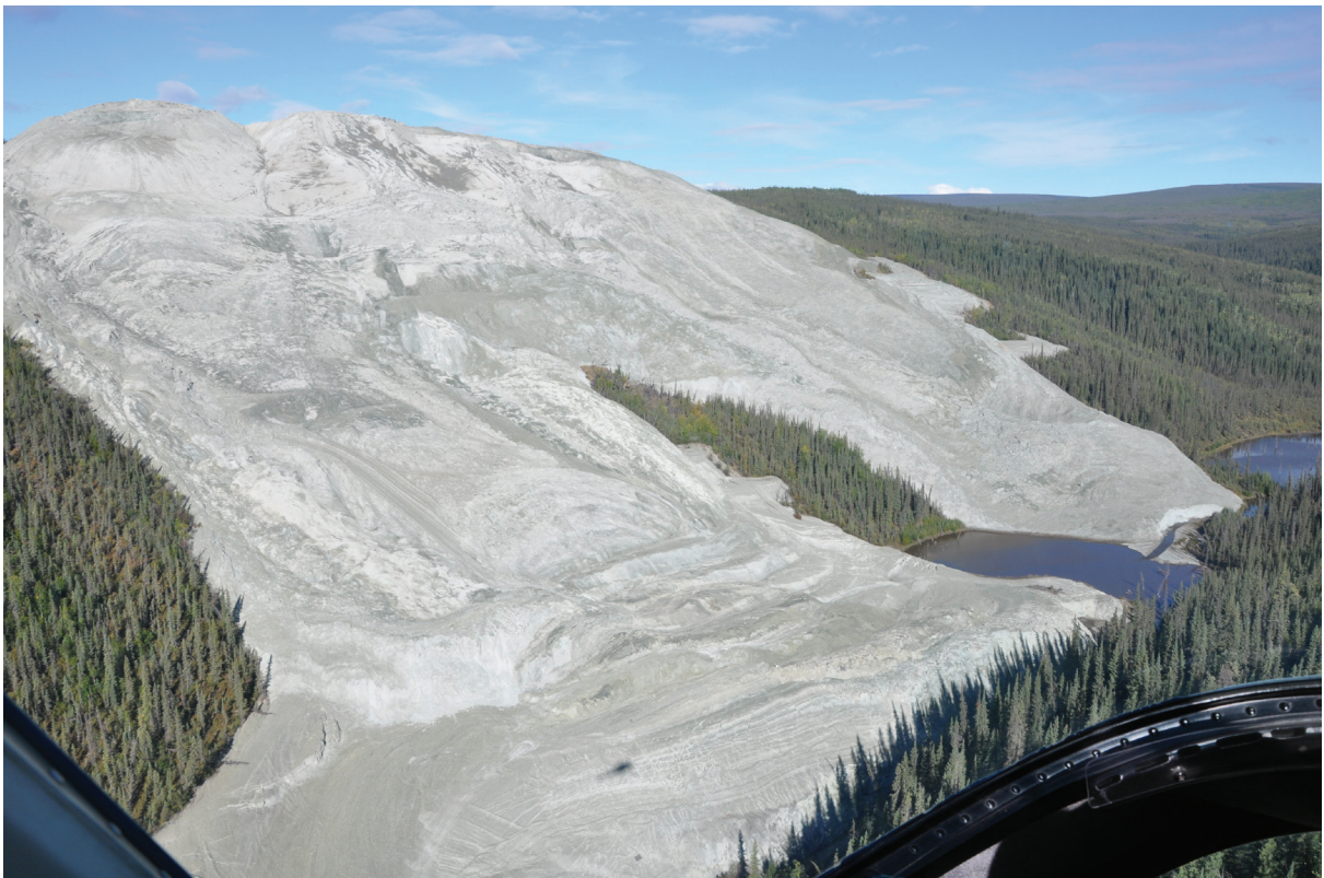
Above: The failed asbestos tailings pile and Wolverine Creek.
