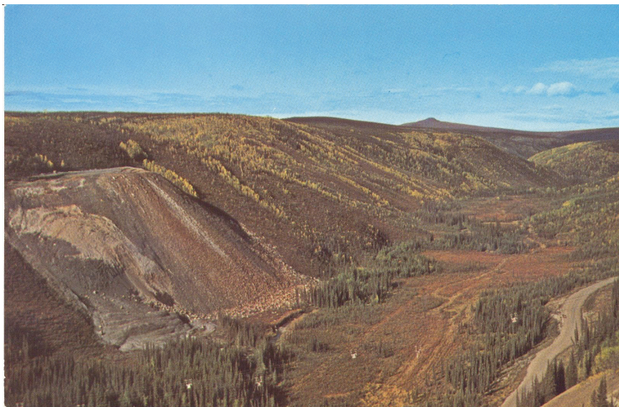
Above: Clinton Creek valley and the waste-rock pile before failure.
